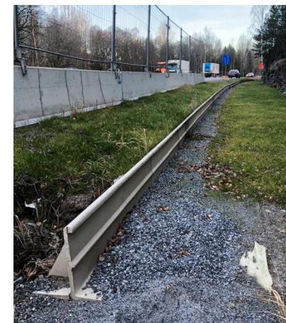
1,3km project in Nacka, Sweden
