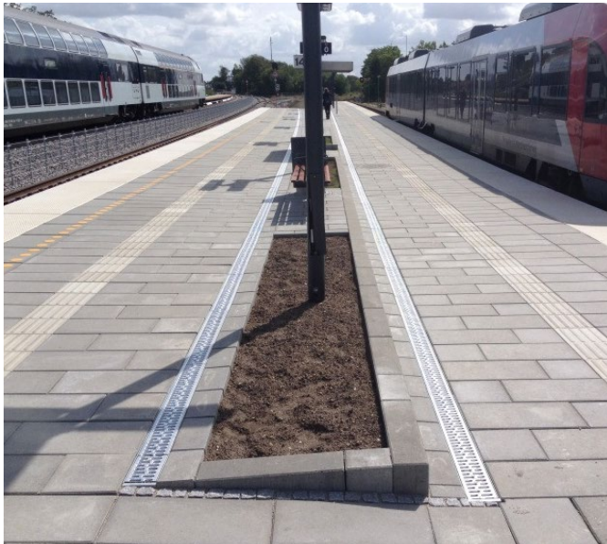
ACO DRAIN® V100S monteret i centerperron
