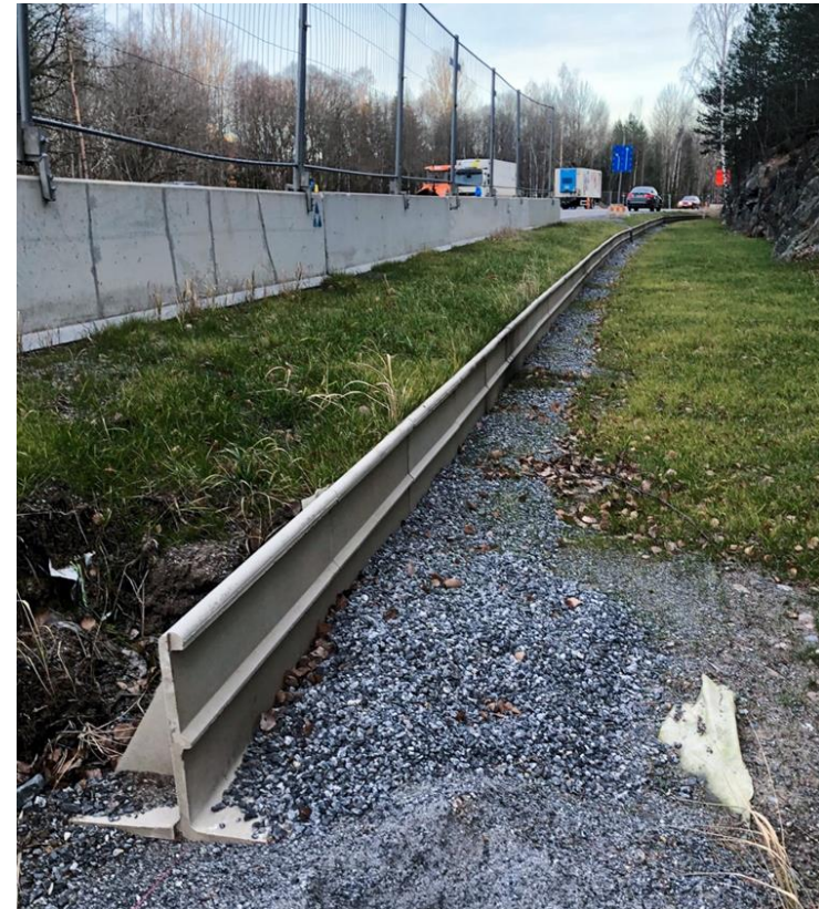
1,3km project in Nacka municipality, Sweden
