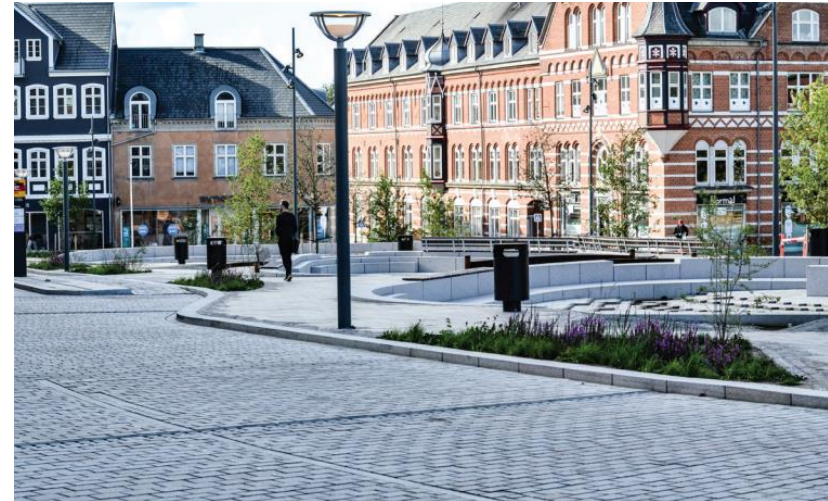
Ringsted, main street and square renovation (Denmark)
